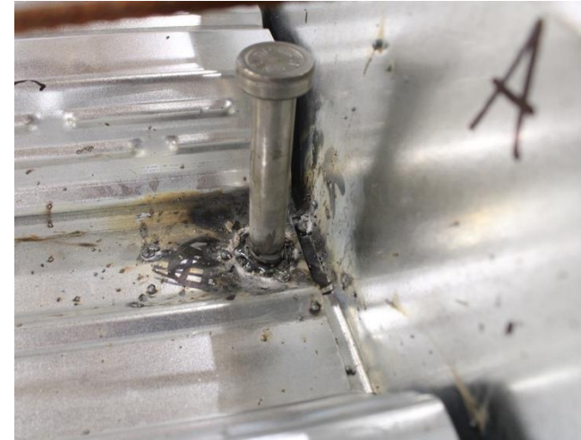
Stud with 1 in. edge distance – Before concrete casting
