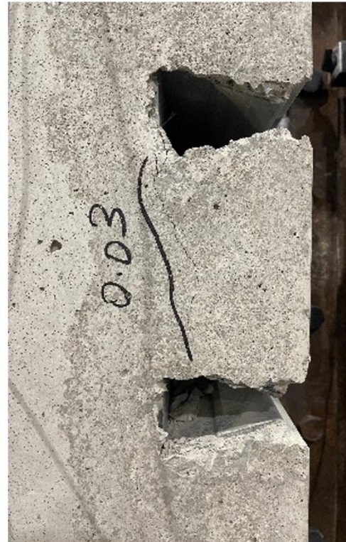
(a) When rib shear crack was formed
