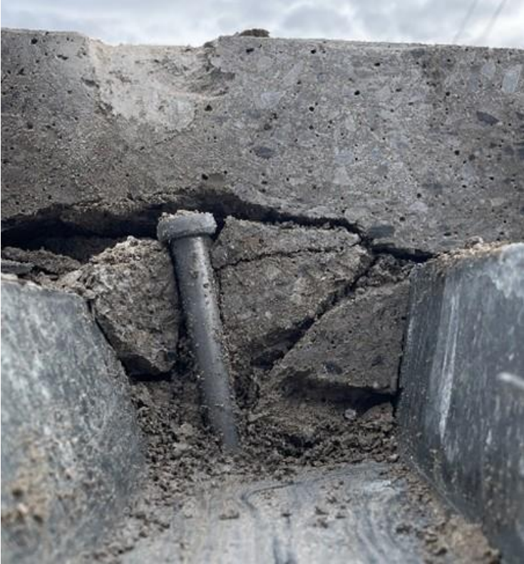
Saw Cut After Testing
