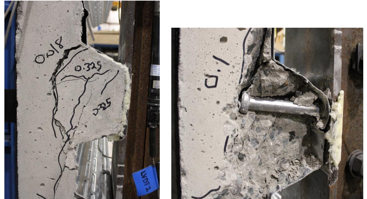
Rib Shear Failure
