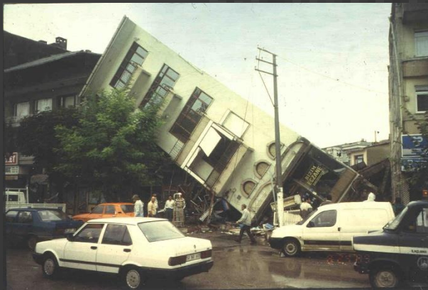
Loss of bearing strength in Adapazari 1999 Koaceli Turkey earthquake
